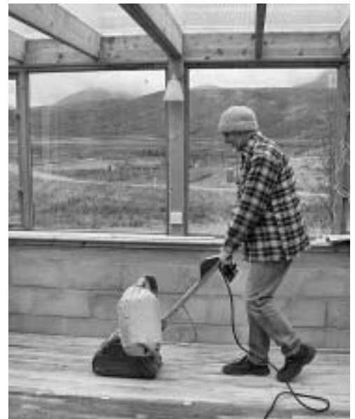
Andy sanding the conservatory floor IY
