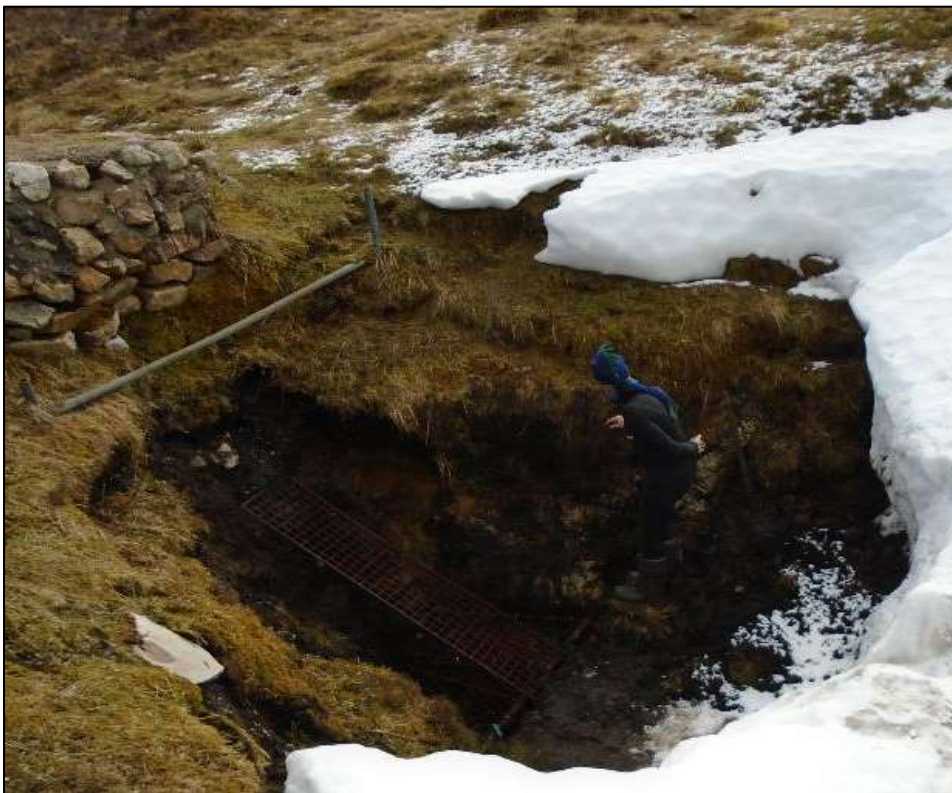
Julian inspecting the slump at the entrance to Rana [JC].
