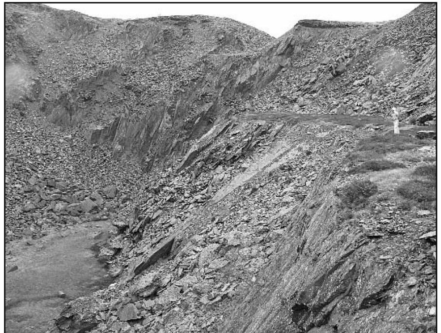
View of North Quarry, with Jim Salvona standing on the bench to the right. The short tunnel ends beyond and behind him.
