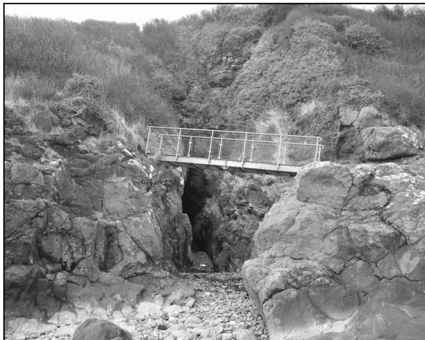
Entrance to Seafield Cave, March 2006, showing footpath bridge.
