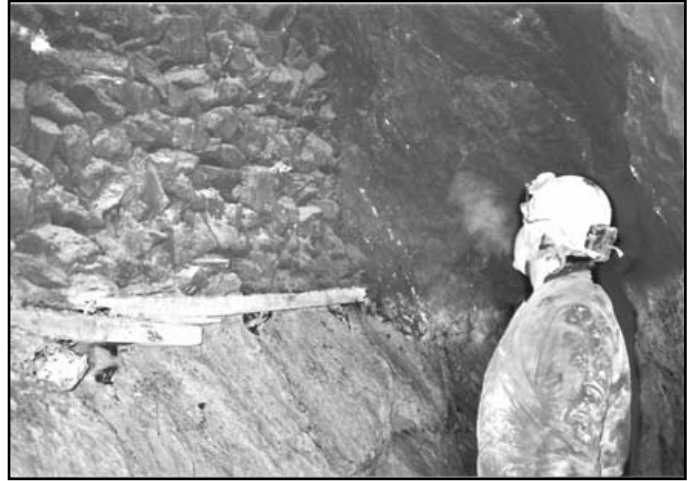
A wall of 'deads' in Parys Mine - possibly a fatal accident just waiting to happen!
