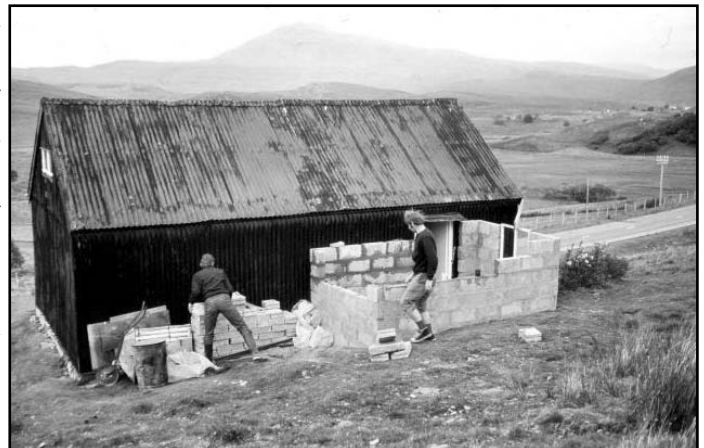
Toilet block under construction, 1976. Left to right: Bob Mehew, Martin Mills.
